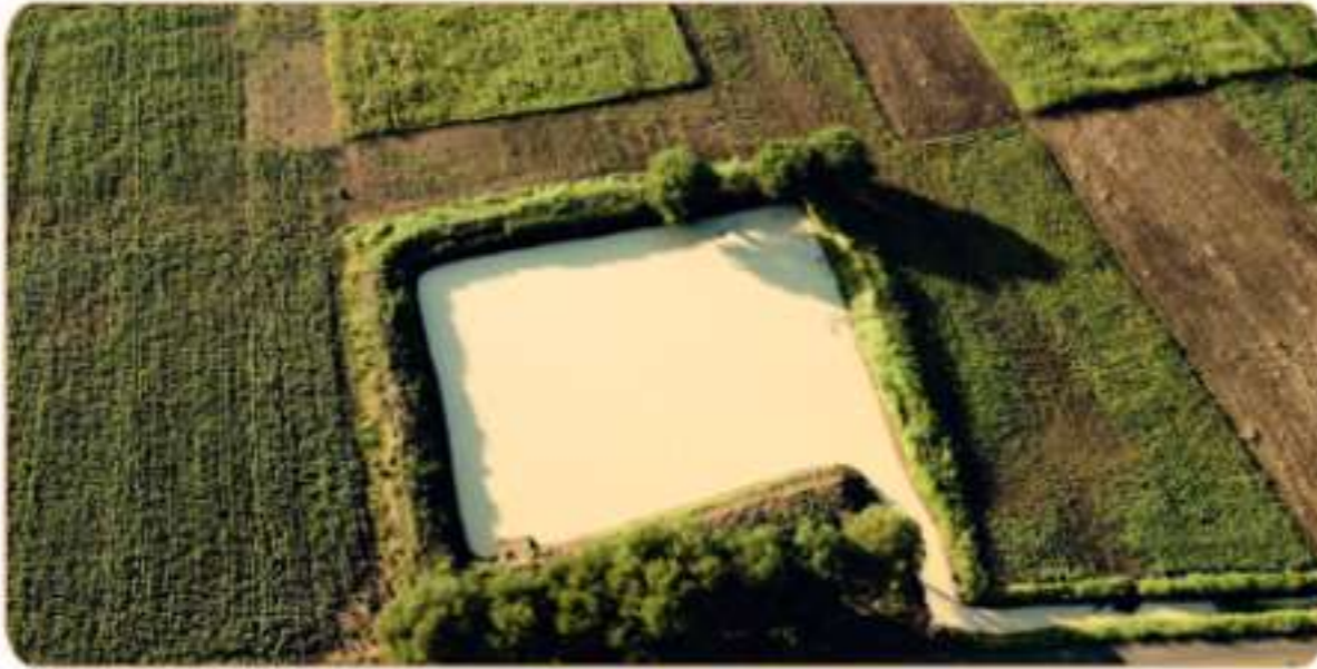
Desilting of Village Pond Sengulam - Virudhunagar District
