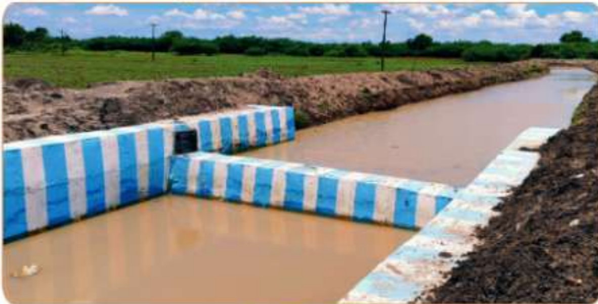
Check Dam Olaipadi - Perambalur District
