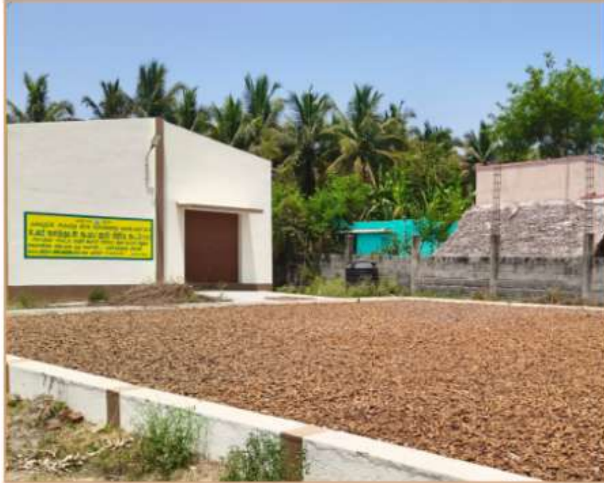
Drying yard with Grading and Sorting hall constructed under Kalaigharin All Village Integrated Agriculture Development Programme - 2023-24 in kanthili, Tirupattur District.
